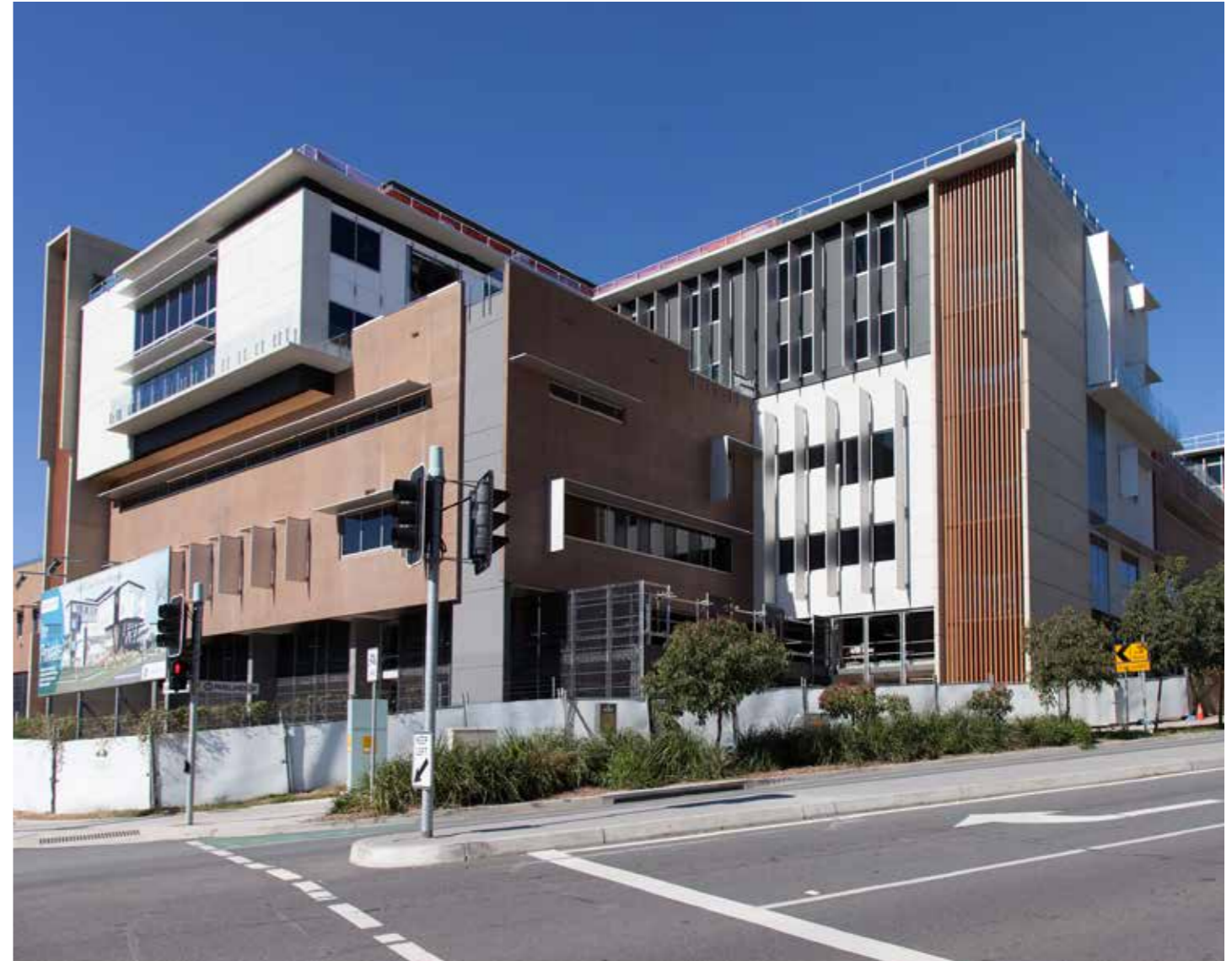
Gold Coast Private Hospital construction in progress
