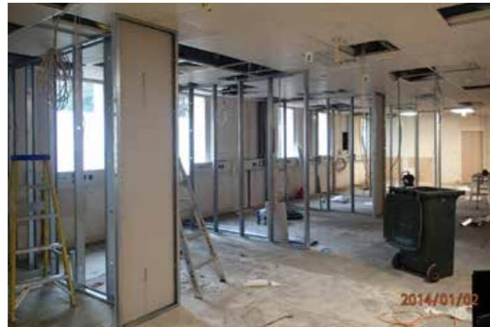
Ashford Hospital Emergency Department during renovation
