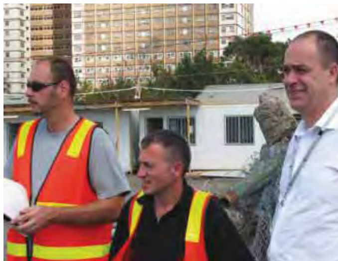
Surveying the site are Luke Perry, Peter Mazzilli and David Rodda
