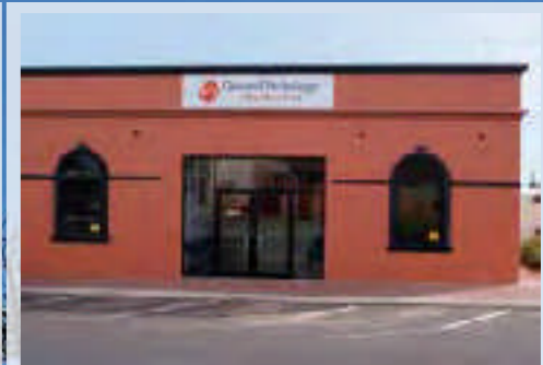
The Kalgoorlie Pathology Laboratory opened in February
