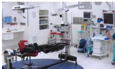
New theatre at Brisbane Private Hospital
