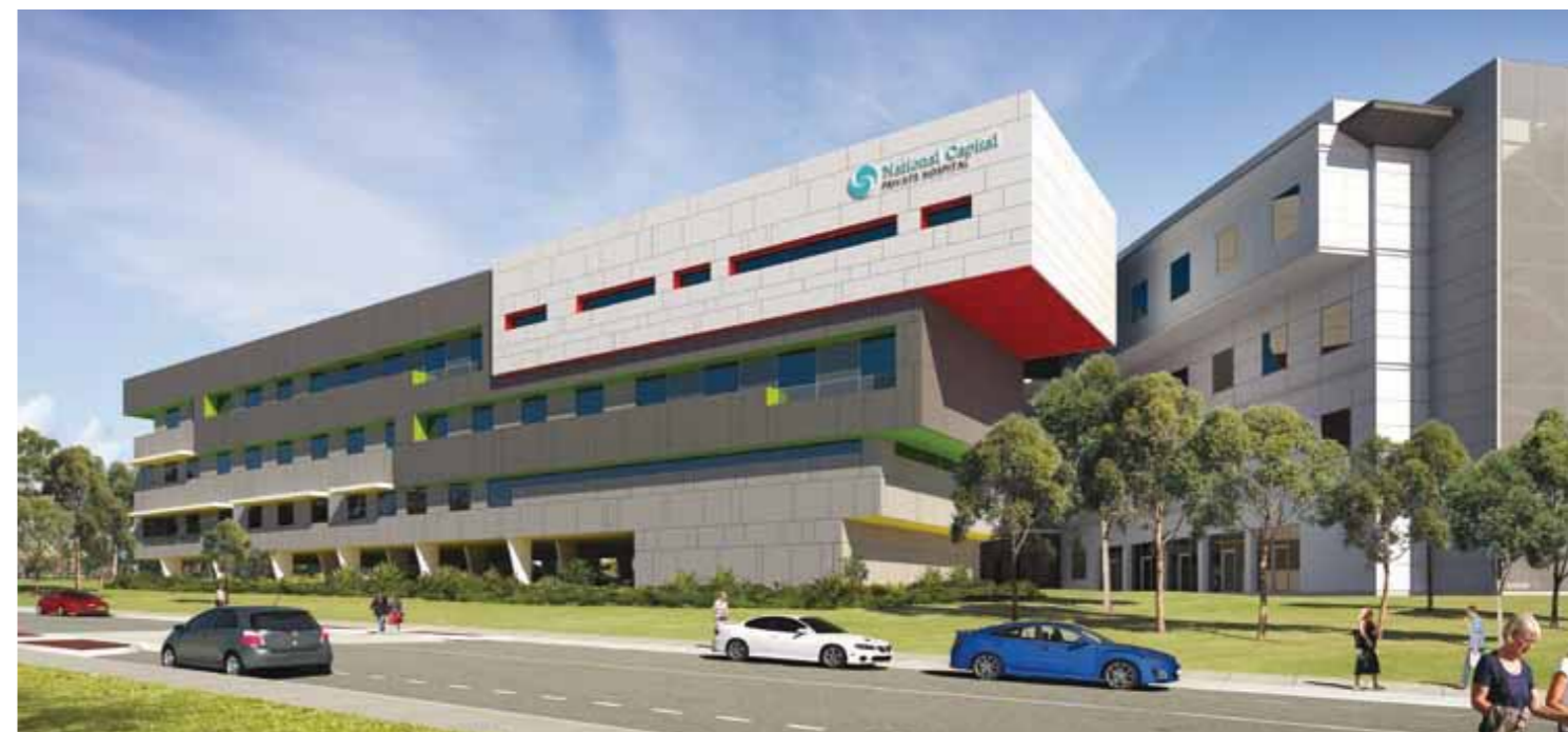
Architect design of the National Capital Private Hospital redevelopment. Construction will commence in 2012
