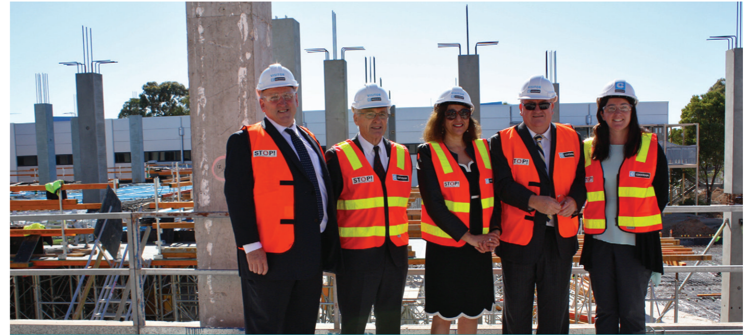
Holmesglen Private Hospital is under construction
